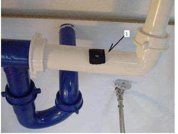
Position the drain saddle in desired location, mark spot. You need to consider available space for drain tubing
