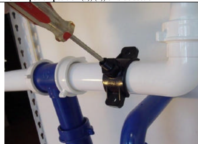
Align the drilled hole in the drain pipe with the drain saddle using a drill bit or narrow screwdriver
