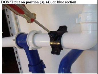
Align the drilled hole in the drain pipe with the drain saddle using a drill bit or narrow screwdriver
