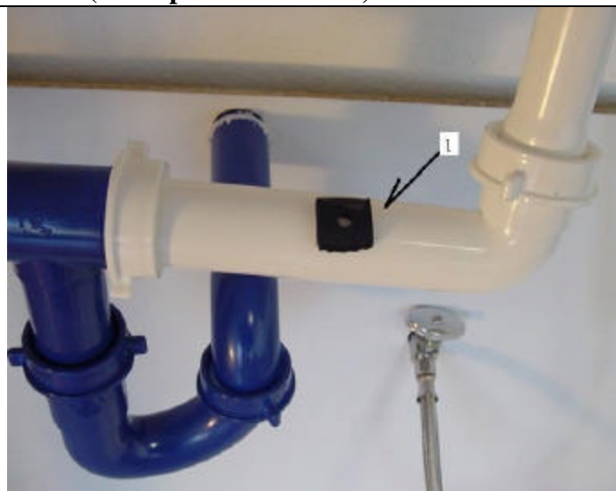
Position the drain saddle in desired location, mark spot. You need to consider available space for drain tubing
