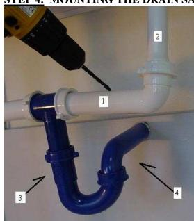
should be installed above the trap and on the horizontal pipe (1) or vertical pipe (2).
