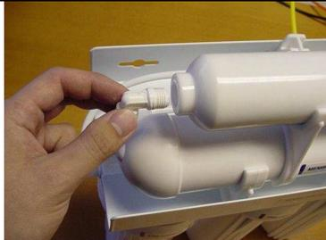
\*unscrew fitting off to replace filter
